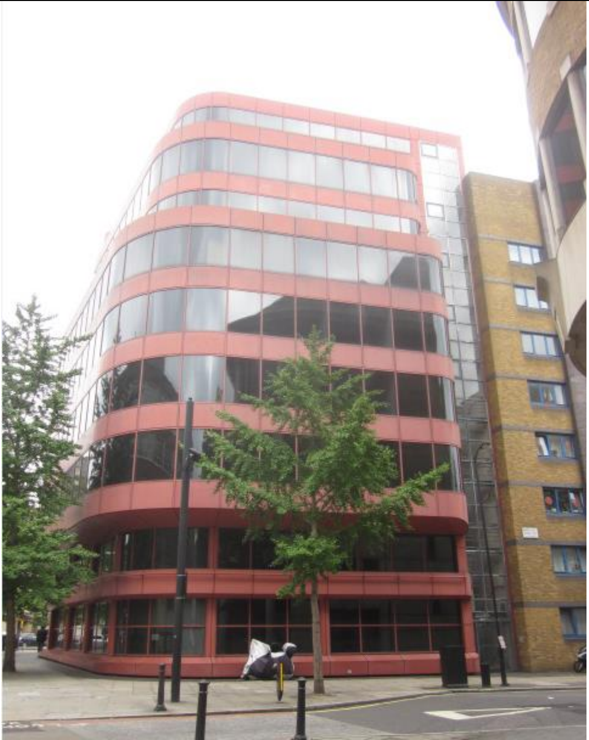
Application site as seen from Harcourt Street and Marylebone Road intersection.
